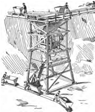
Fig. 8. Operation of Portable Gravity Mixer.
